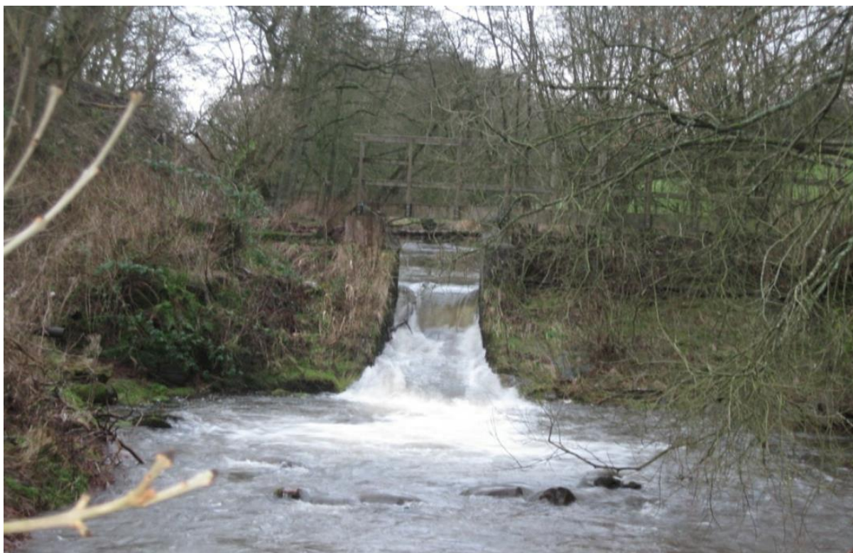
Figure 1: Gateside Mill Weir prior to removal
