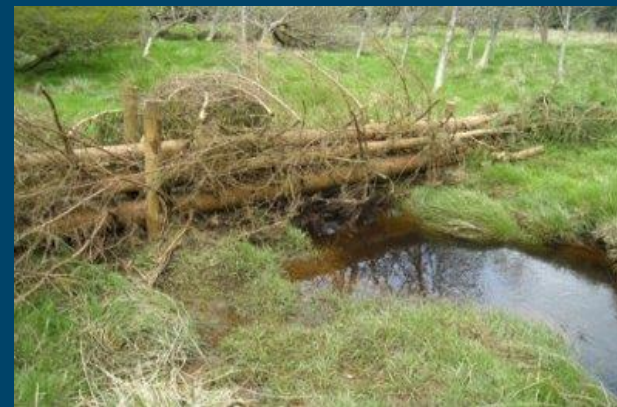
install high-flow log restrictors
